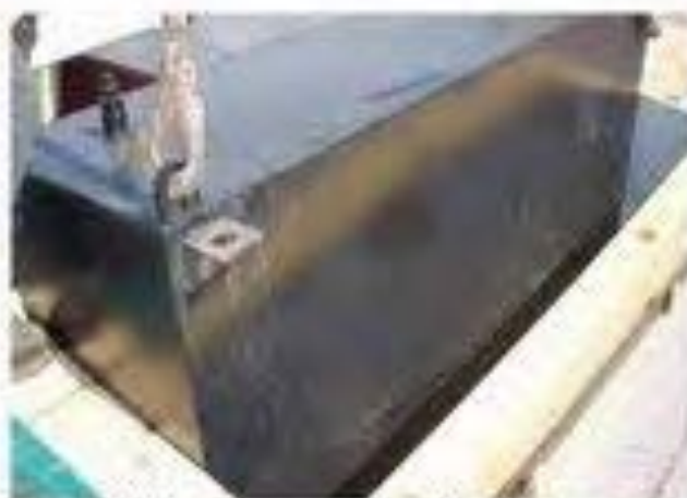
Tight squeeze for diesel tank
