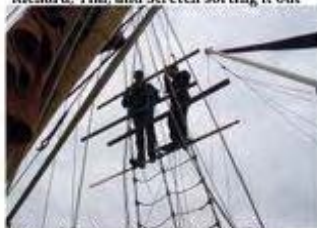
Up the rigging making ratlines
